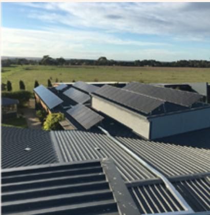
Solar panels have been installed at Alan David Lodge.
