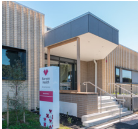
The new Renal Services building opened in mid-August.
