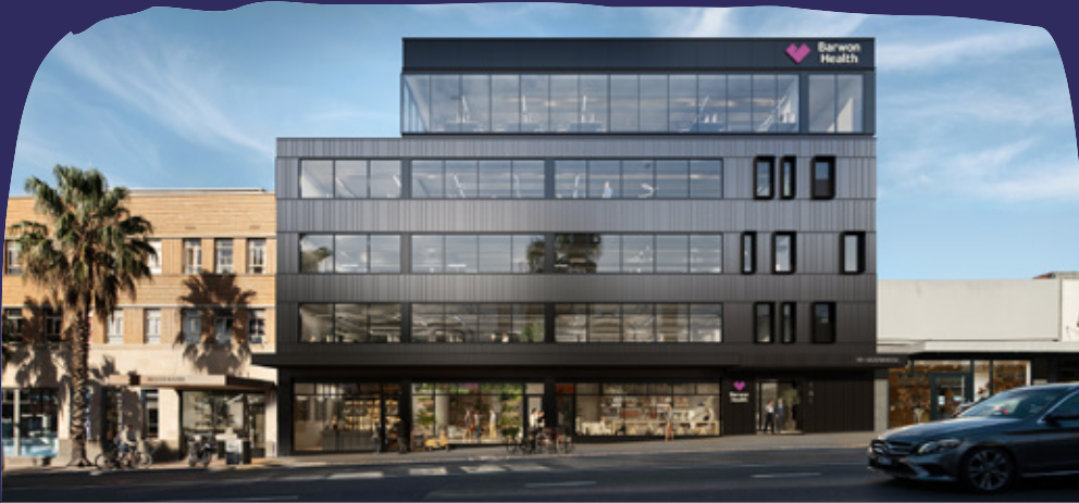
The Lived Experience Network provided valued input to the project team designing the Mental Health Hub under construction in Moorabool Street (artist's render pictured).
